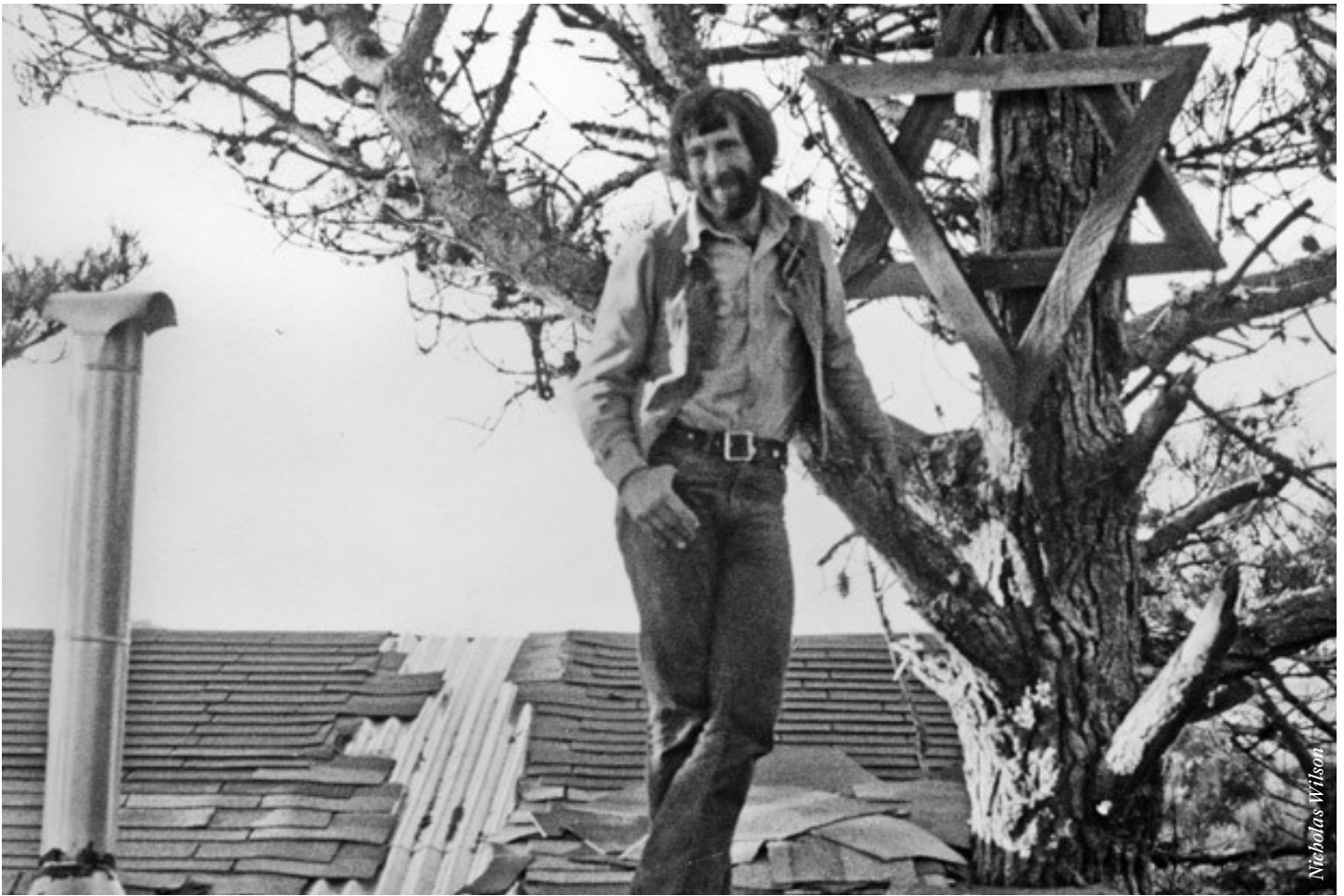
Stephen Anapolsky on the roof of the Mendocino Coast Jewish Community Centre, circa 1968.
